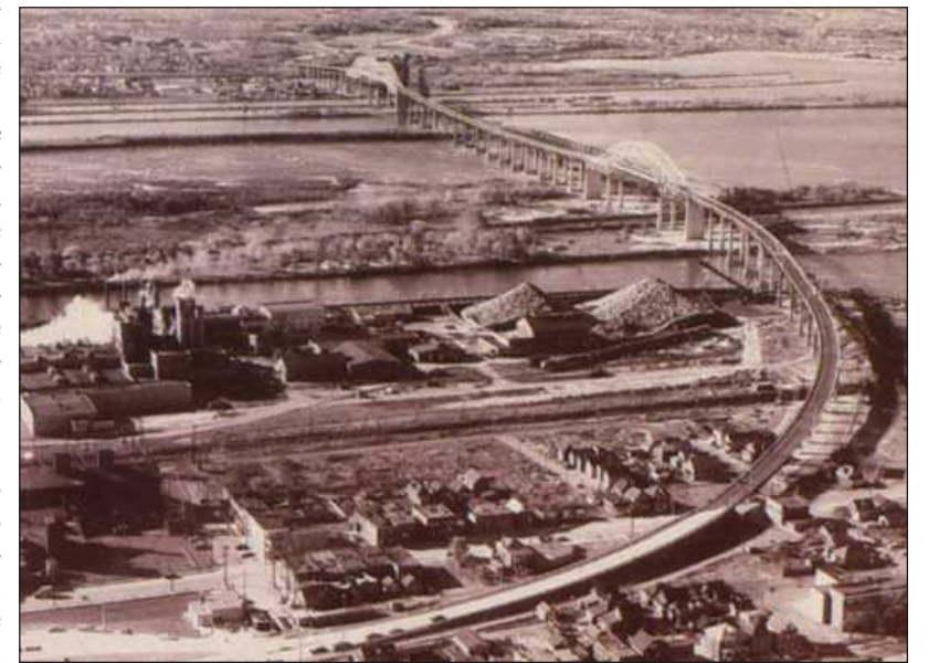
AN AERIAL VIEW of the International Bridge from the U.S. side. A dip in the span in between the arches using shorter piers was a construction cost-saving measure. Photo credit: International Bridge Authority
