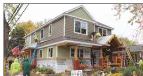
SHEETMETAL WORKERS Local 80 Instructor Sam Velez, with the angle square at right, shows a group of third-year apprentices working at the Wencel house how to make a cut of metal roofing. The apprentices include (l-r) Nathan Landry, Matt Wardrop, Evan Smiecinski and Alex Bastien. The Wencel house, at left, has a new second floor to make more room for their adopted children.
